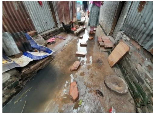
Figure 11: Rainfall induced waterlogging.
