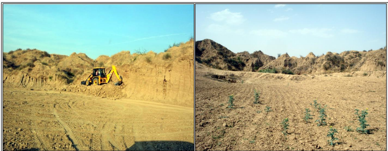
Plate 1. Massive land levelling in the study area and conversion of ravine land into agricultural land
