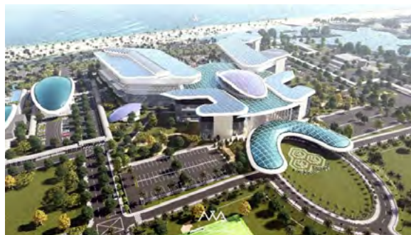
Figure 5. Pusat Rehabilitasi PERKESO Terengganu (under construction, 2027)
