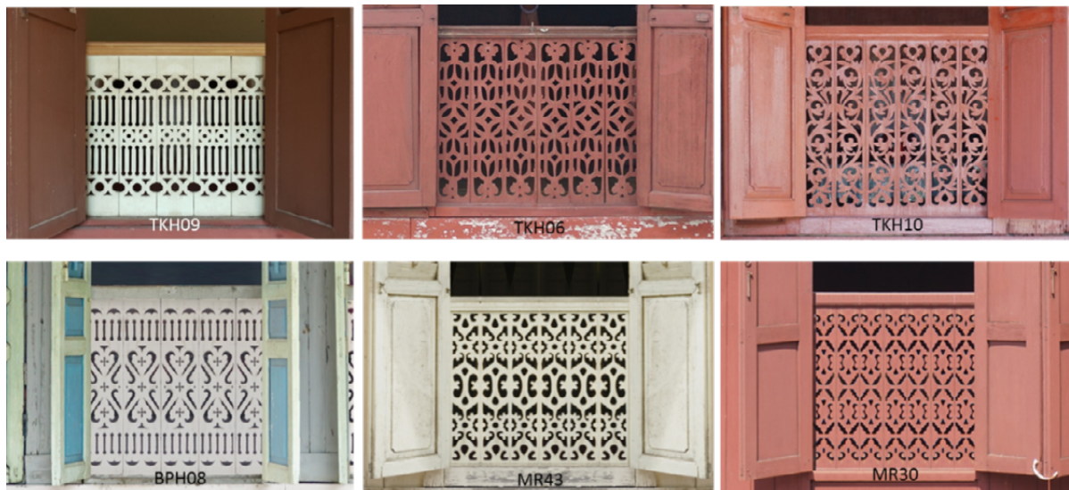
Figure 8 Jerjak tingkap panel uses a pattern that is beautiful standing alone but becomes even more beautiful when it meets and is sandwiched closely with other panels with the same pattern design. The term for the discovery of this pattern is named as “ rapat bertaut .”
